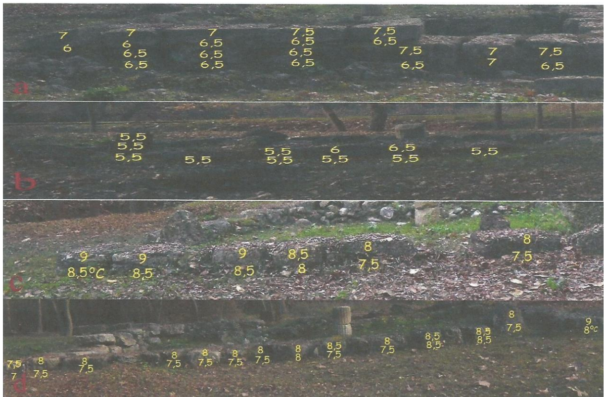
Figure 8 IR thermometer measurements, wet conditions, Asklepios temple, a) north side, b) east side, c) south side, d) west side
